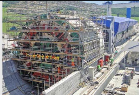
Largest tunnel boring machine (TBM) to date. 15.7m diameter, Sparvo, Italy, 2011.
